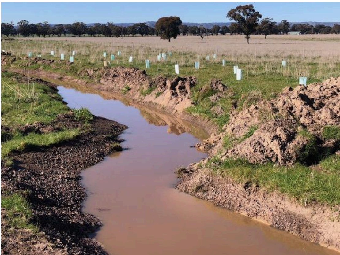
Image 3. Adding more life through revegetating new contour channels in the landscape on Coolwoola Plains. Source: The Winter-Irvings.
