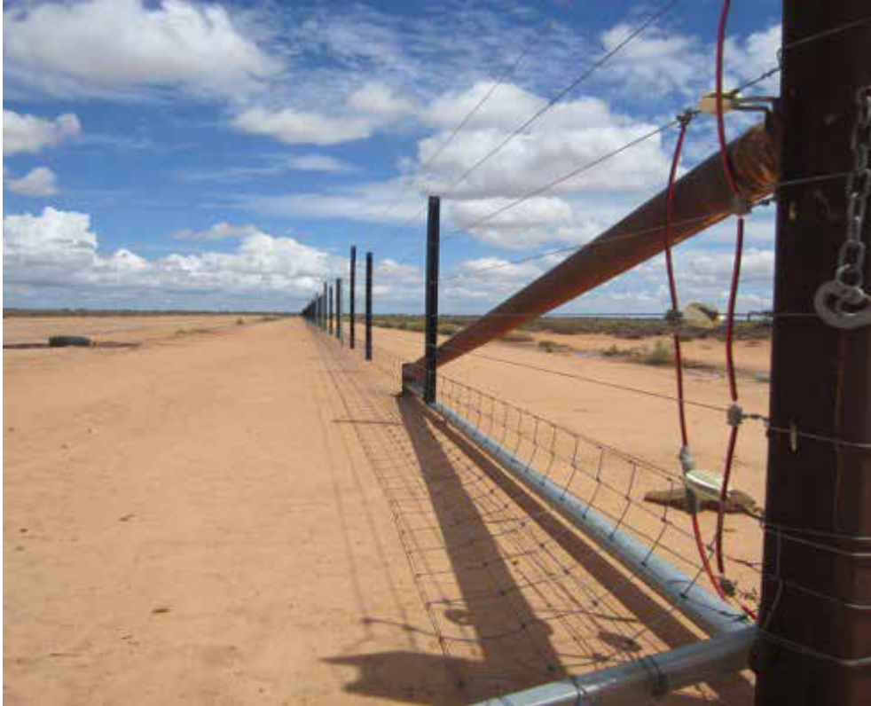
Figure 9: Kangaroo-proof fence: extra height wire supported by fewer posts; mesh apron to prevent kangaroos pushing under the bottom wire; two electrified mid height wires powered by solar panels.
