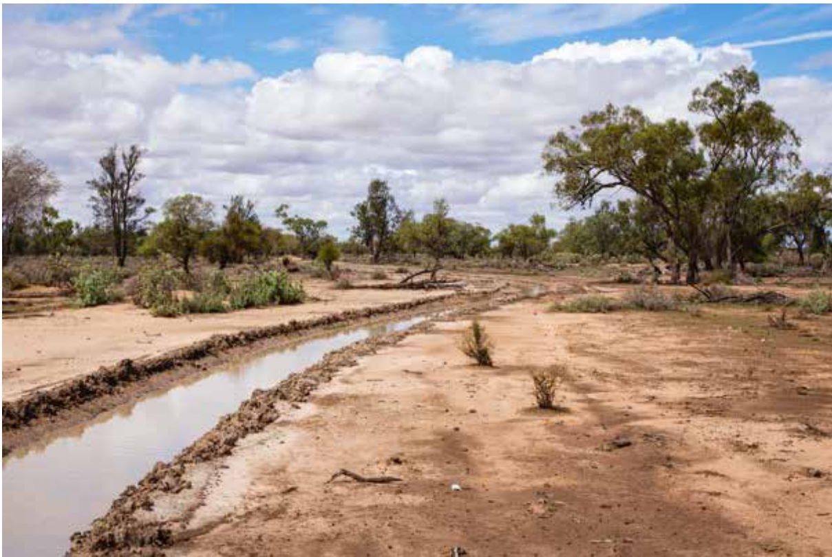
Figure 6: One of the four bore drains that together used to carry away around 250 ML/year of surplus water.
