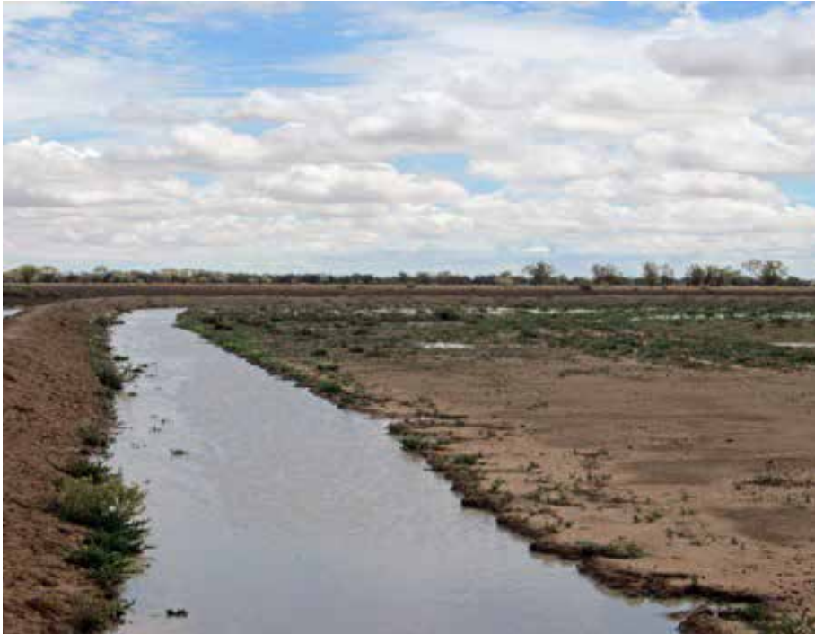
Figure 3: A horseshoe pond bank with water ponding in the trenches either side of the bank and across the surface. Regenerating vegetation is evident within the horseshoe.
