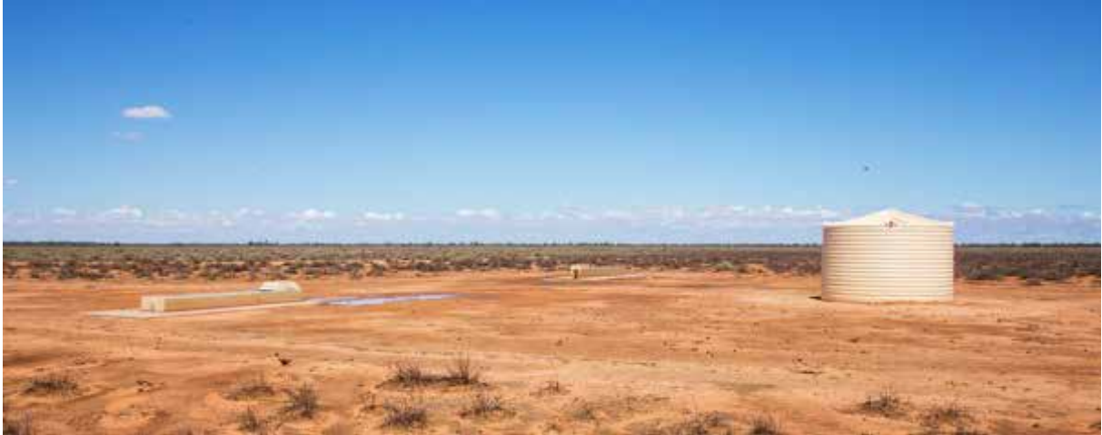
Figure 7: Tank and troughs that have replaced free-flowing artesian bores.
