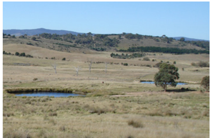
To minimise evaporation, dams were made as deep as possible with small surface areas
